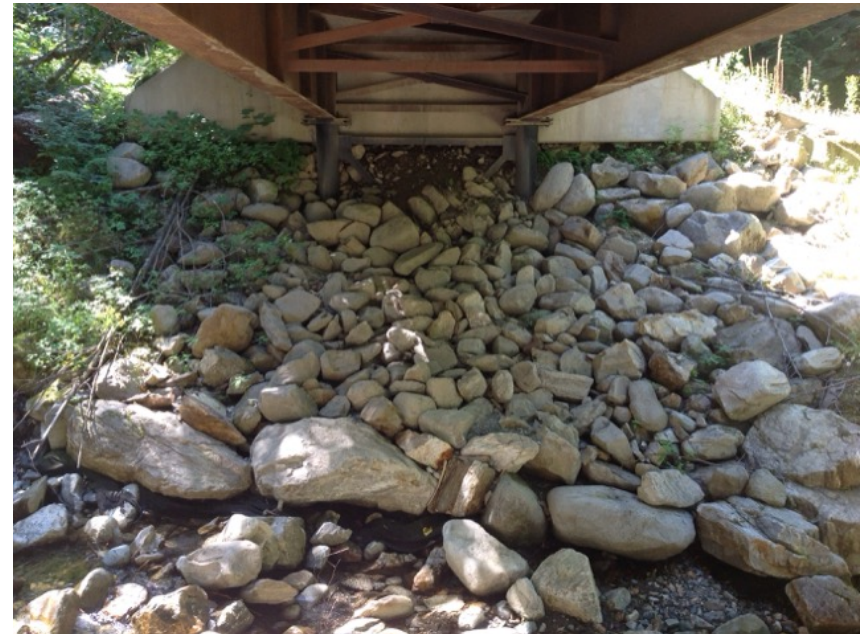
Left Bank Abutment when facing downstream
