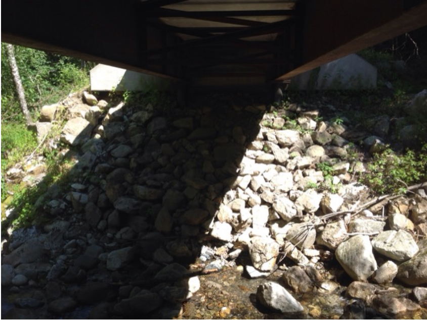
Right Bank Abutment when facing downstream
