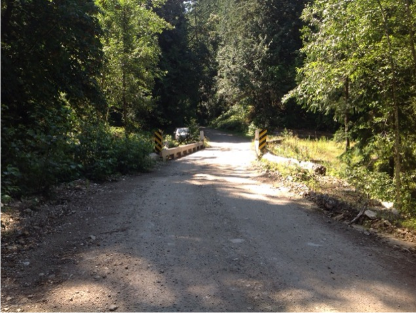
Approach from Right Bank when facing downstream
