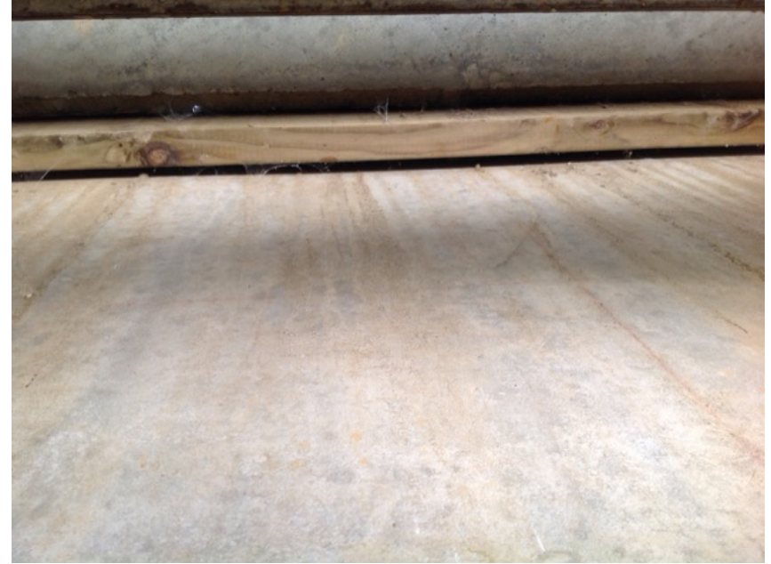
treated 2x4 to help hold fill in place on right bank
